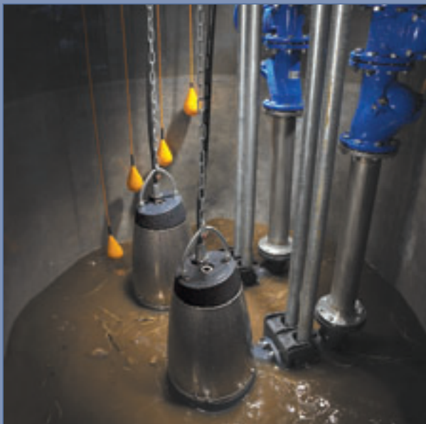
Submerged installation on auto-coupling with guide rails When installed on an auto-coupling system, the pump automatically connects to a base unit fixed to the bottom of the pump pit.
